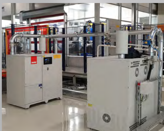
Centrale turbine HE
