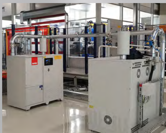
Turbine centrale HE
